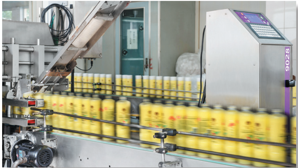
9028 inkjet printer installed on bottling line.
